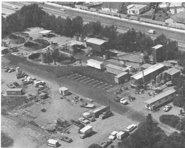
Figure 2. The 1 MGD pilot plant
