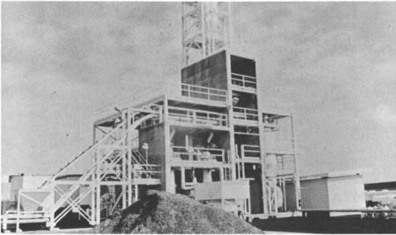
Figure 1. Albany, Oregon biomass liquefaction PDU
