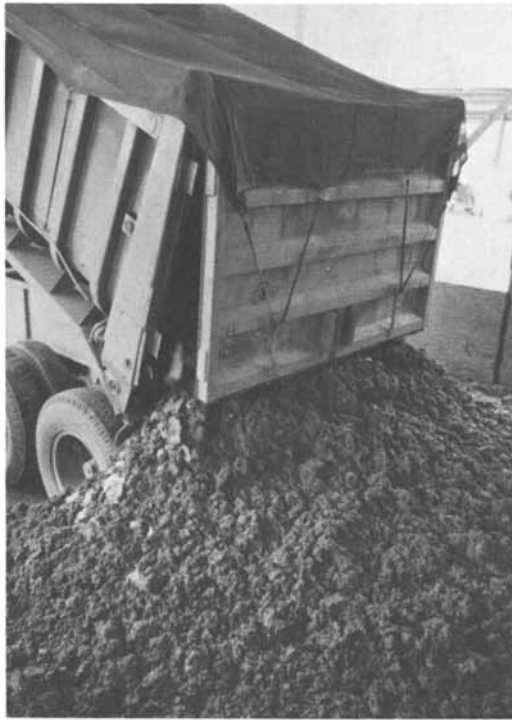
Figure 4. Sludge cake at dumping station
